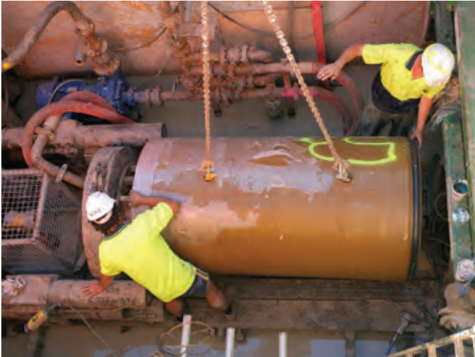
Micro-tunnelling in action.
