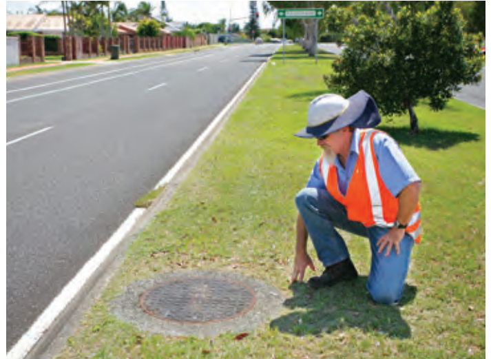
A restored pipeline construction site, with only a manhole visible.
